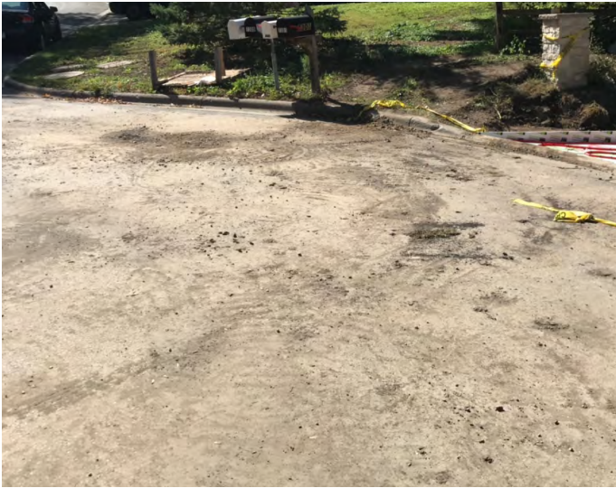
The image above shows tracking of sediment onto a street from a 2022 construction site, which violates District permit rules.
