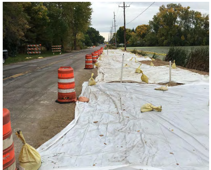
Covering exposed soils during road work reduces the risk of erosion into Duck Lake (fall 2021).
