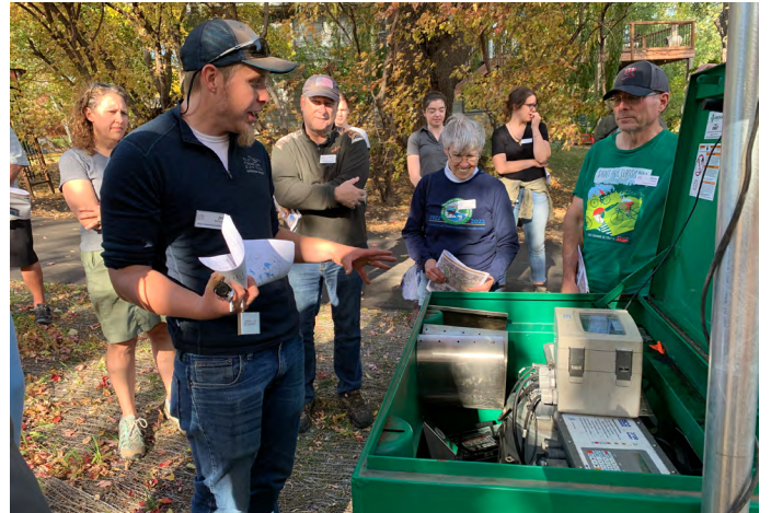
Josh Maxwell, Water Resources Coordinator, explains operation of the automated sampling unit for the Kraken filtration units for the Rice Marsh Lake Stormwater Management Project (Stop 3).
