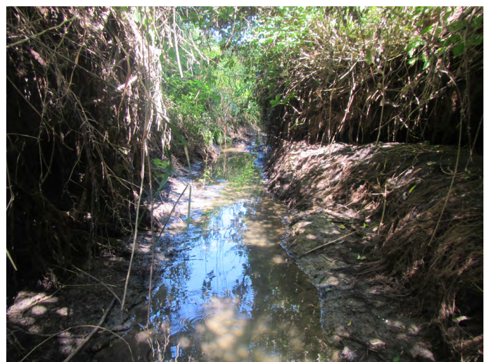
Images of eroding banks and incised channel of Riley Creek - Reach 4 (R4) from 2022.
