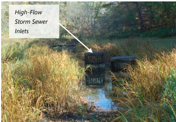
B. High-flow inlets to a storm sewer along an existing stream corridor (Source: RWMWD)
