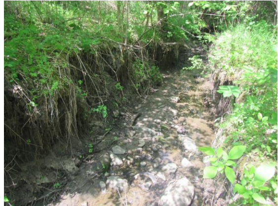
Increasing volumes of stormwater runoff erode streams (Bluff Creek shown here). This is due to both the runoff from impervious surface as well as runoff from green space where compacted soils increasingly shed stormwater.
