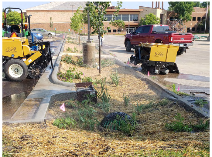
Photo of tree trench installation for the St. Hubert Opportunity Project.
