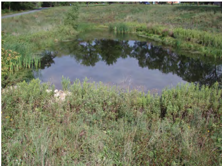
Park Pond (2009) (receives storm flows from Subwatershed 3)
