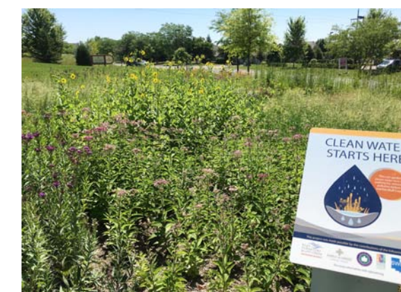
The garden captures, filters, and slows down stormwater runoff from the church's 1.4-acre parking lot. It removes pollutants like phosphorus and sediment before they enter nearby Bluff Creek.
