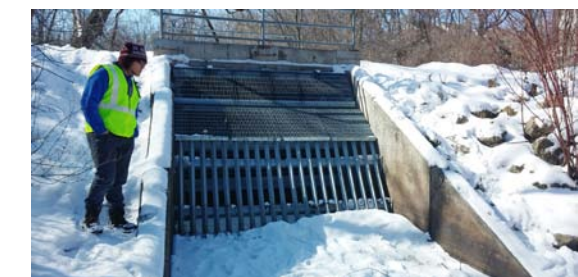
This barrier keeps carp from moving back downstream. It is put in after the carp have migrated upstream in the spring.
